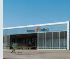
Ameco A380 Hangar Peking, China
