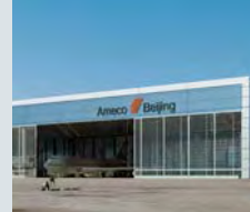
Ameco A380 Hangar Peking, China
